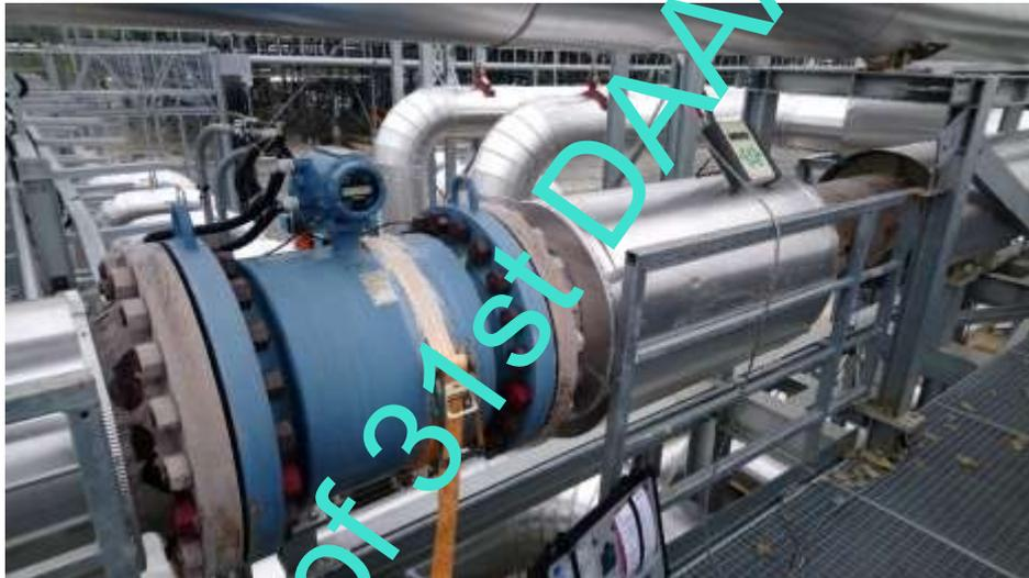
Fig. 4. Measurement point at the separator outlet pipe
