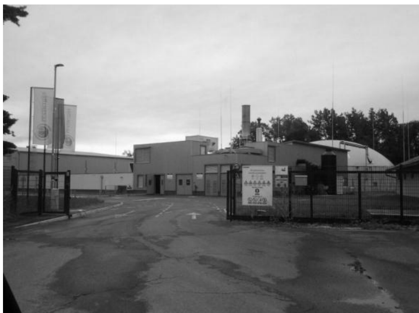
Fig. 1. Biogas plant Drazenci
