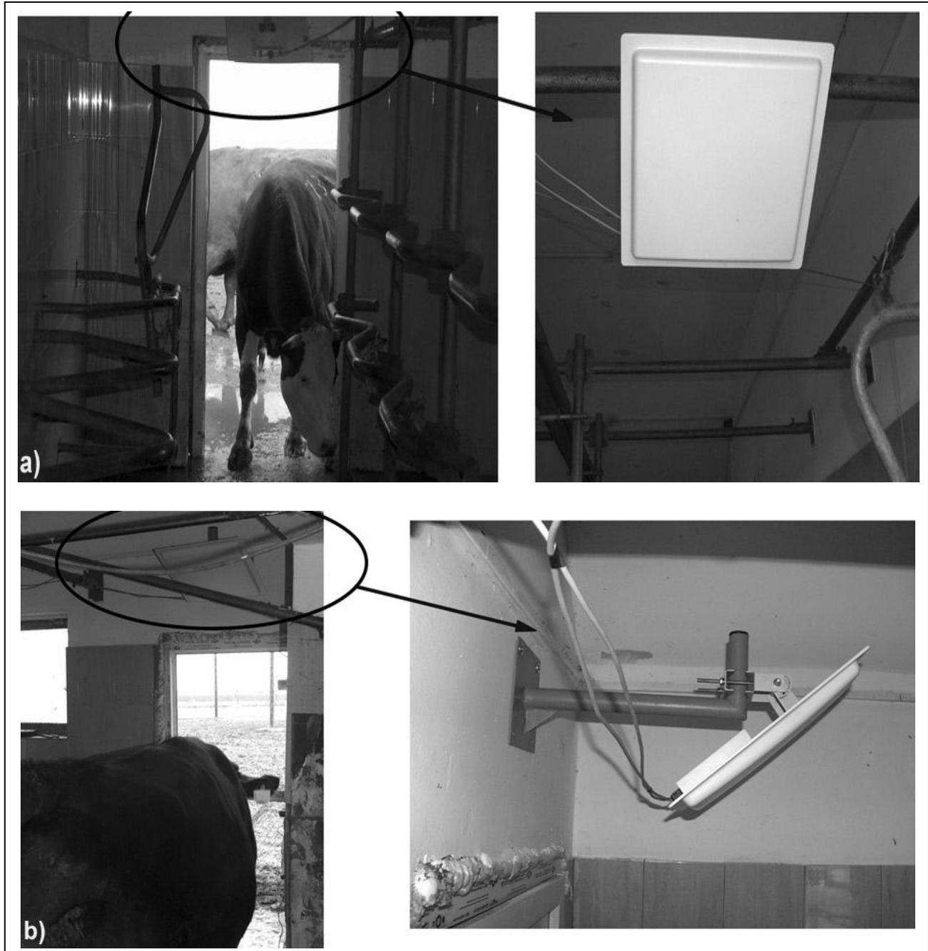
Fig. 9 a). RFID reader at the entrance to the milking facility; b) RFID reader at the exit from the milking facility
