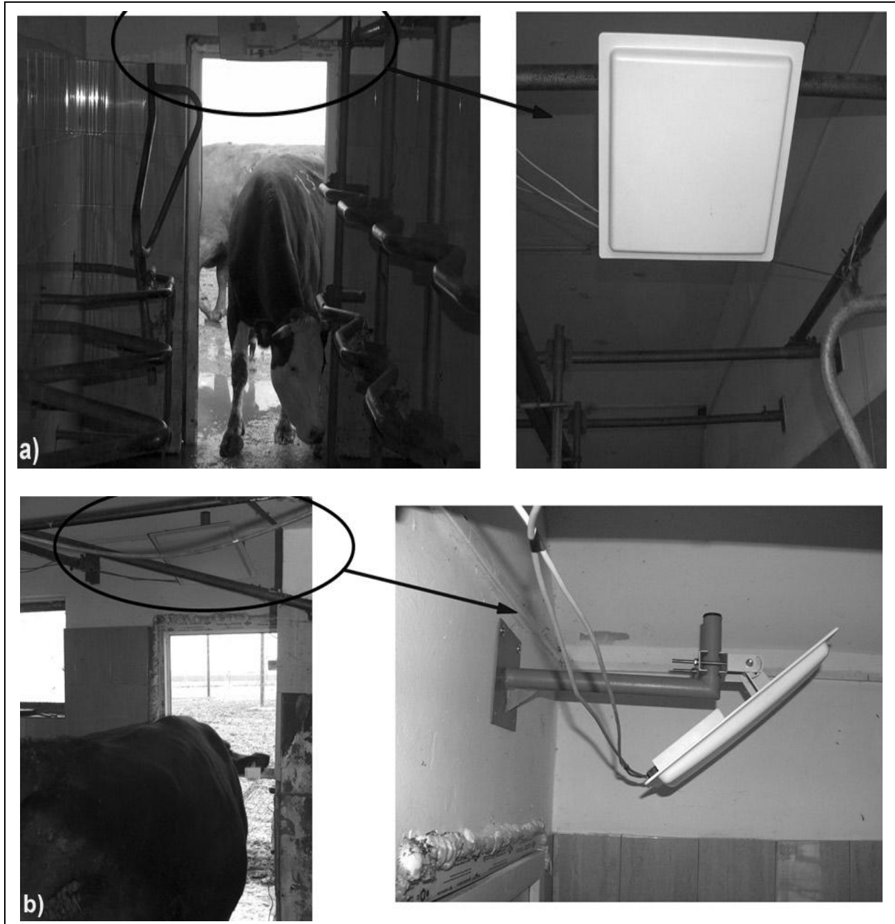
Fig. 9 a). RFID reader at the entrance to the milking facility; b) RFID reader at the exit from the milking facility
