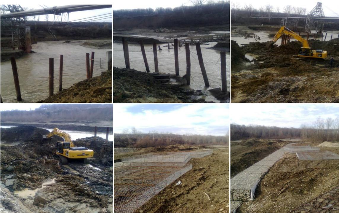
Fig. 1. From top left are shown the works of securing oil pipelines  $\text{Ø}10 \frac{3}{4}$  "Ø12" Ø14" Cartojani-Ploiesti.
