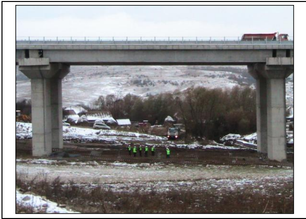
Fig. 2. Viaduct on the A3 Transylvania Highway
